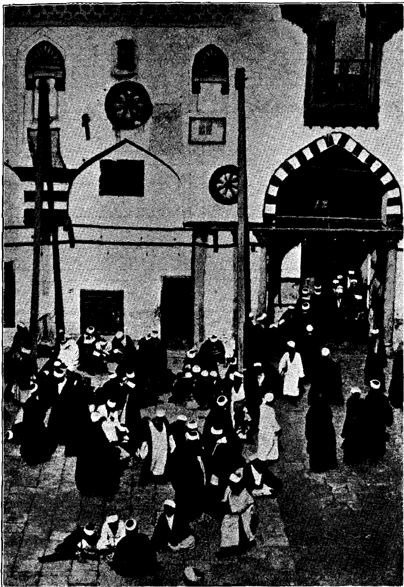
INTERIOR OF MAIN COURT, EL AZHAR UNIVERSITY, CAIRO. Showing the dilapidated condition of the building.
